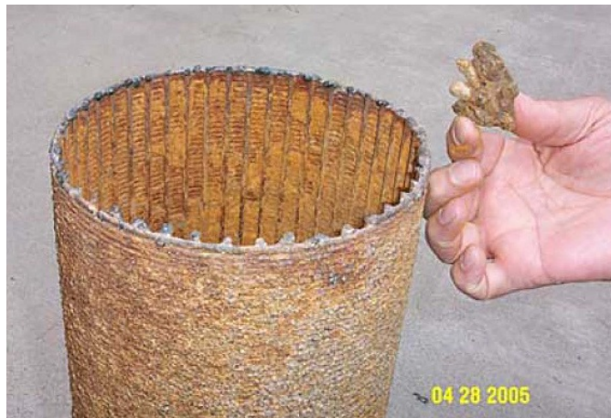
Incrustation on the well screen
